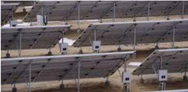
Figure 8: Example of a typical string inverter
